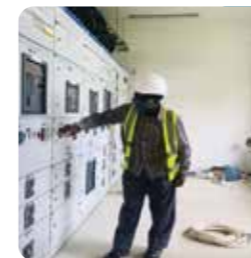
Commissioning of Main LV Panelboards at CCBRT hospital project
