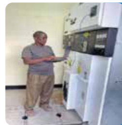
HT Switchgear commissioning at Arusha Technical college-Kikuletwa Moshi to Shinji
