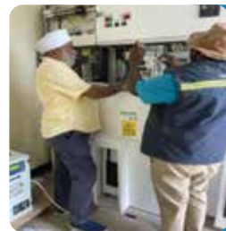
Installation of HT Switchgear at Arusha Technical college-Kikuletwa Moshi
